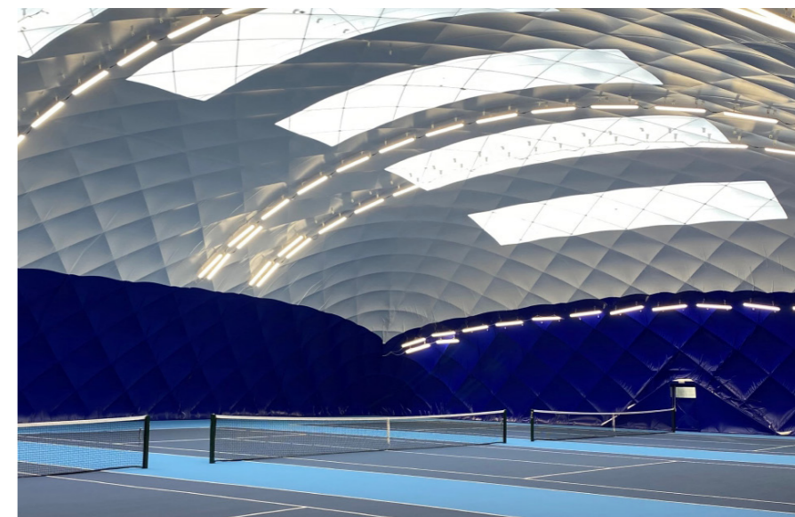
"Air dome", externally & internally (above)
