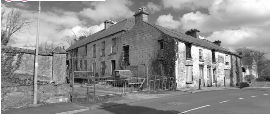
2 & 3 Existing heritage buildings.
